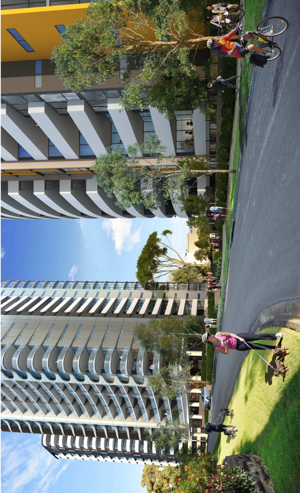
VIEW FROM GAY STREET LOOKING SOUTH
